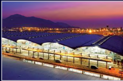
Hong Kong International Airport
